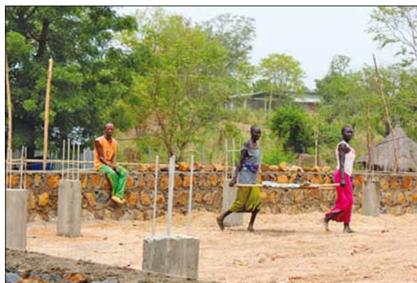
Constructing the chapel at St Frumentius Anglican Theological College.
